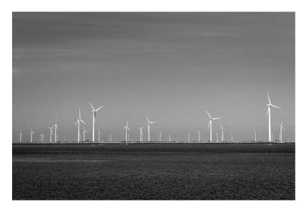
The mean power output of the wind farm is 696 MW, which is enough power for 580 000 homes.
